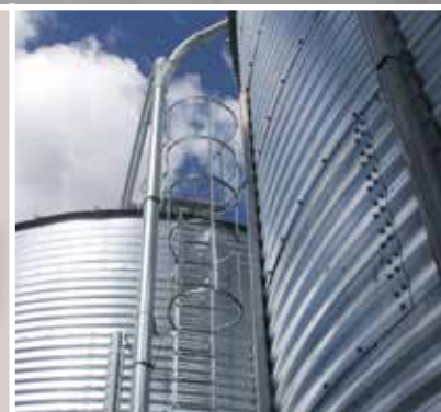
Pipe assembly for filling outdoor steel silos.
