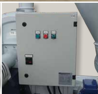
Control cabinet for automatic starting/stopping the motor.
